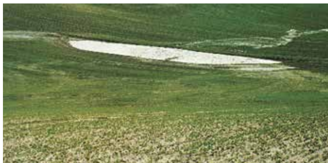
A sediment basin temporarily holds sediment on property where construction is underway and in other places to keep sediment and debris out of reservoirs, lakes, and streams.
