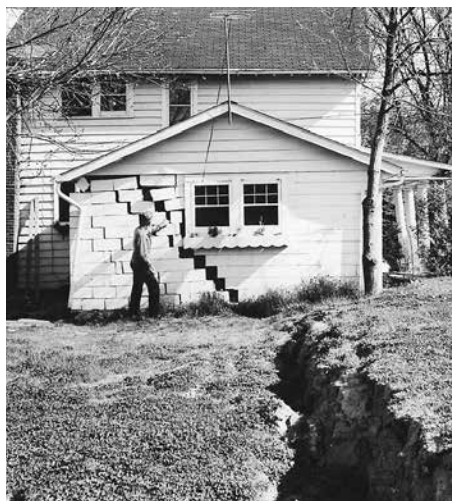
Paying attention to soil interpretations can help builders and landowners avoid this kind of disaster. Soil slippage and swelling caused this house to break apart.
